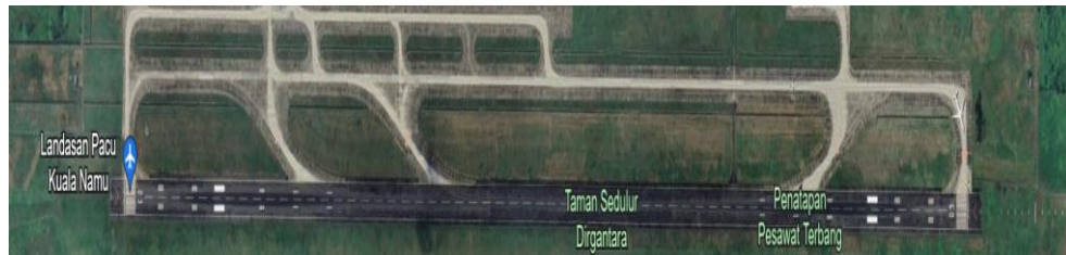
Gambar II. 1 Taxiway Bandara Internasional Kualanamu (Sumber : Google Earth )
