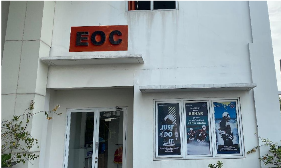
Emergency Operation Center
