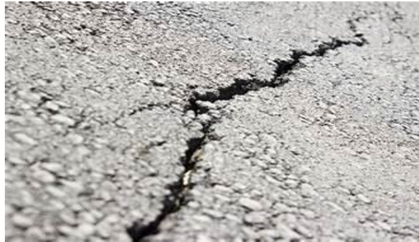
Gambar II. 21 Retak diagonal
