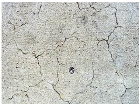
Gambar II. 26 Scaling/Map crack/Crazing
