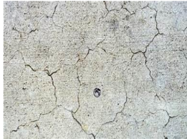
Gambar II. 26 Scaling/Map crack/Crazing
