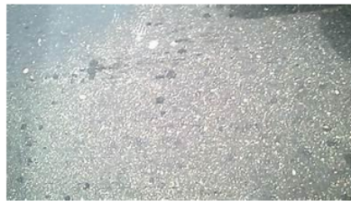
Gambar II. 17 Agregat licin
