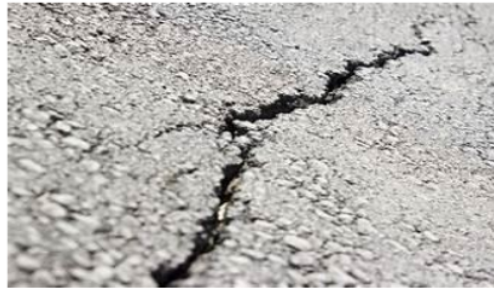
Gambar II. 21 Retak diagonal
