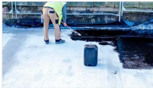
Gambar II.2 Penerapan *waterproofing coating*
