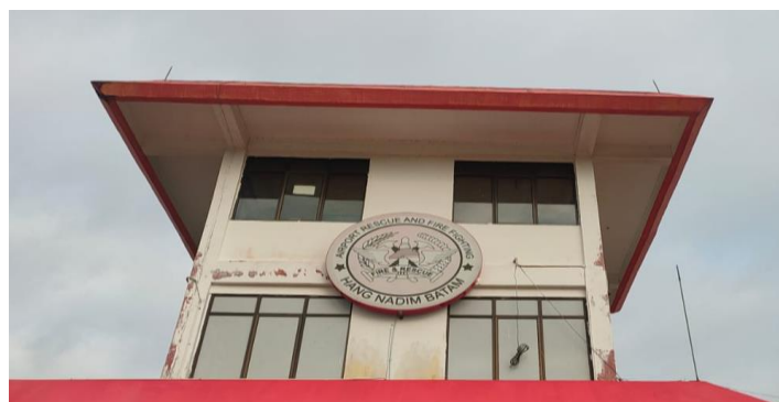
Gambar II. 2 Tampak luar watchroom Hang Nadim
