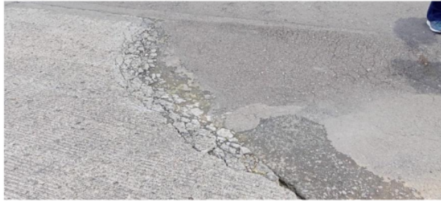
Gambar IV.2 Alligator Crack
