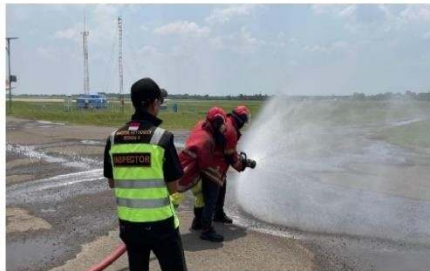
Pengujian Handline Operation
