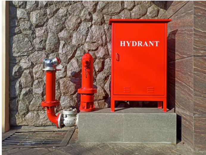
Gambar II. 10 Outdoor hydrant box
