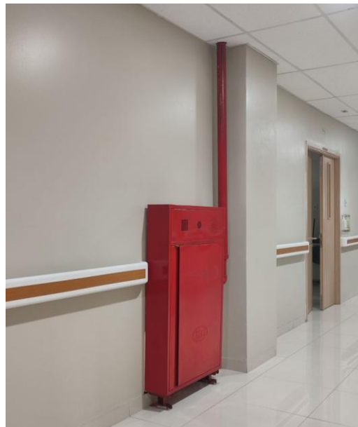
Gambar II. 9 Indoor hydrant box
