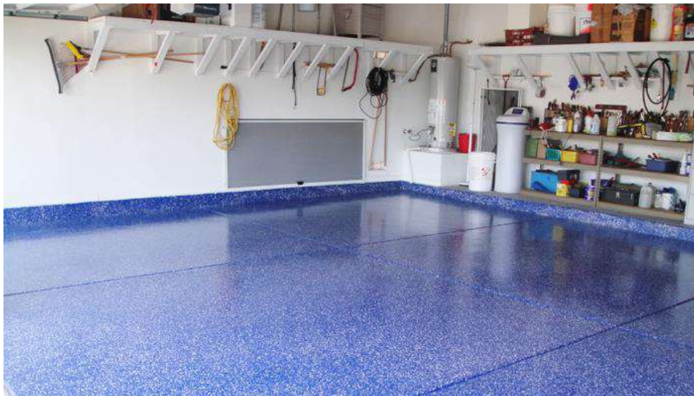
Gambar II.1 Lantai Epoxy (internet)
