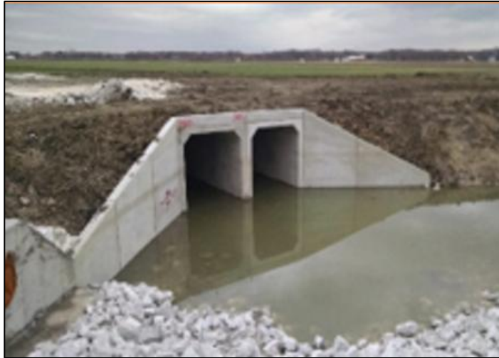
Gambar II. 4 Tampak Melintang Box Culvert Sumber: (Saidah dkk, 2021)
