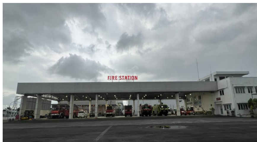
Gambar 2. 2 Fire Station Bandar Udara Ahmad Yani Semarang Sumber : Fire Station Bandar udara Semarang
